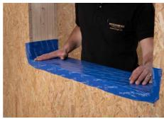
> Thanks to its high extensibility, Ampacoll® Sillskin can effortlessly be installed in the corners. The result is a continuous one-piece cover.
