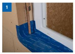
> After the window has been installed, the window sill base is stuck to the outside of the window frames with Ampacoll® Sillskin.
