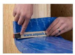
> Schematic diagram for timber construction (left) and application example of Ampacoll® Sillskin (right). Side overlap: DE  $\geq$  10 cm; AT  $\geq$  6 cm.
