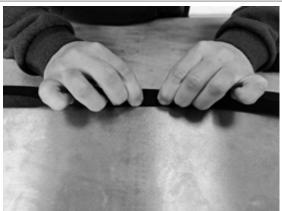
Check that the seal is correctly inserted in the groove.
