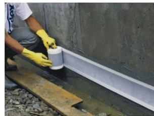
3. Overcoat VANDEX CONSTRUCTION JOINT TAPE with a second coat of VANDEX BB 75 E (minimum layer thickness is 2,0 mm) and smooth the surface with damp brush.
