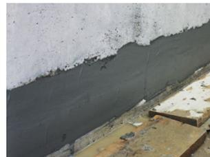
4. Finished state: Provide appropriate protection of the tape if required.
