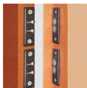
Double electrical contacts between leaf and doorframe
