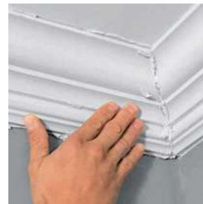
Apply special Jointing Adhesive to the cross-section of the profile. Push the cornices tight against each other until glue squeezes out.
