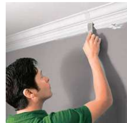
Remove excess glue. Fill the joints and nail holes with a fine filler using a spatula.
