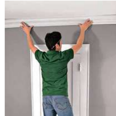
Mark the installation line on the wall and ceiling using a pencil or a chalk line.
