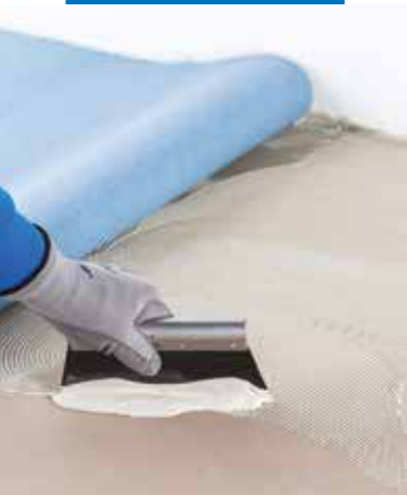
Aplicarea Ultrabond Eco TX1
