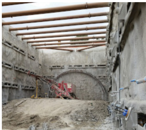
Shotcrete with Mapefibre MB 65
