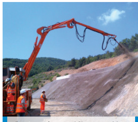
Entrance of a tunnel Shotcrete with Mapefibre MB 65
