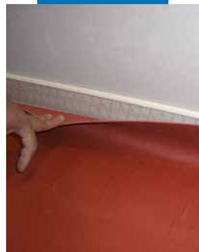
Forming a fillet shell using Mapecoat
